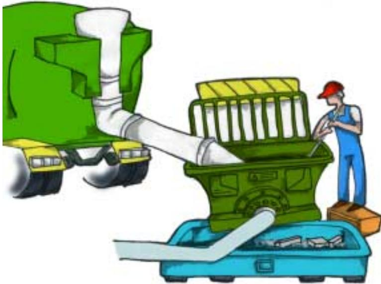
The unit can then be removed to allow excess wet concrete to be handled without contaminating the stormwater system.
